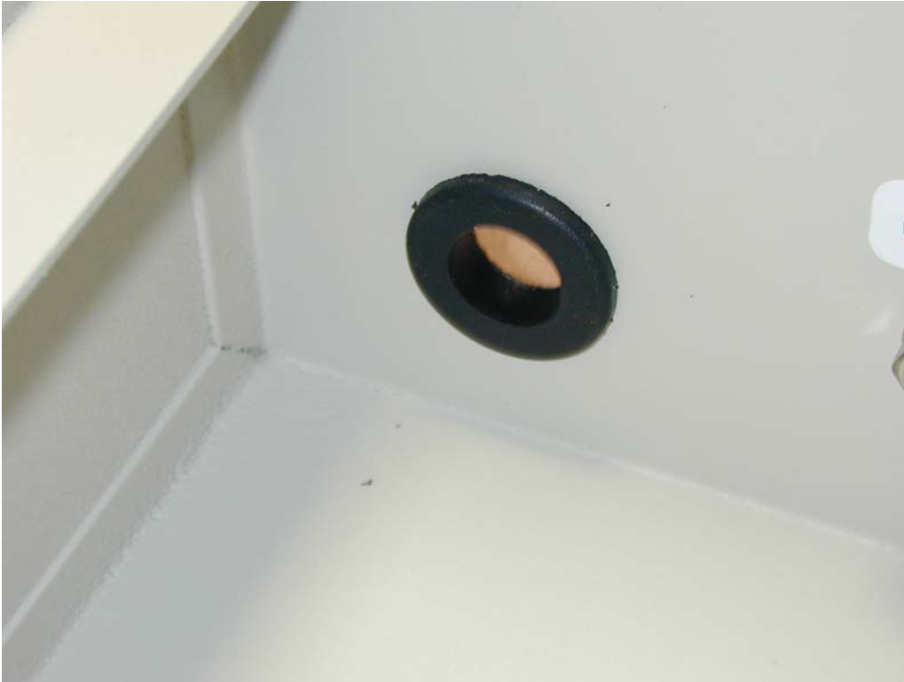
Figure 2 - Grommet Insertion
